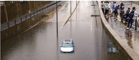
A vehicle partially submerged in a waterlogged underpass after heavy rainfall, near Sabarmati riverfront in Ahmedabad on Thursday PTI
