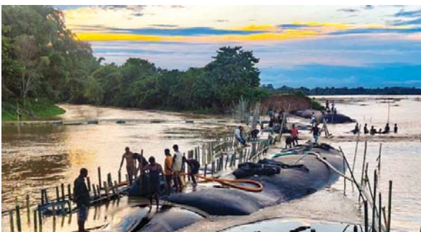
People gather on geo-tubes amid embankment repairs as part of the Assam Flood Response in Jorhat
