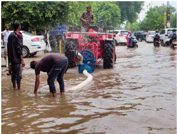
Workers use a tractor-mounted water pump to drain accumulated rainwater from a waterlogged road following heavy rainfall in Gurugram, Haryana on Saturday PTI
